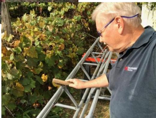
Next I moved on to refurbishing the tower sections I have. I needed to wire brush the old paint off as much as could be done. Then I painted them with a brown Rustoleum rust primer. Then with an exterior coat.
