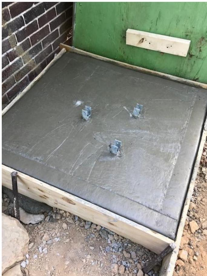
After the cement was poured it was time to strip some of the upper bracing off and skim the surface with a trowel to smooth it out and to put on a rounded edge to the block.
